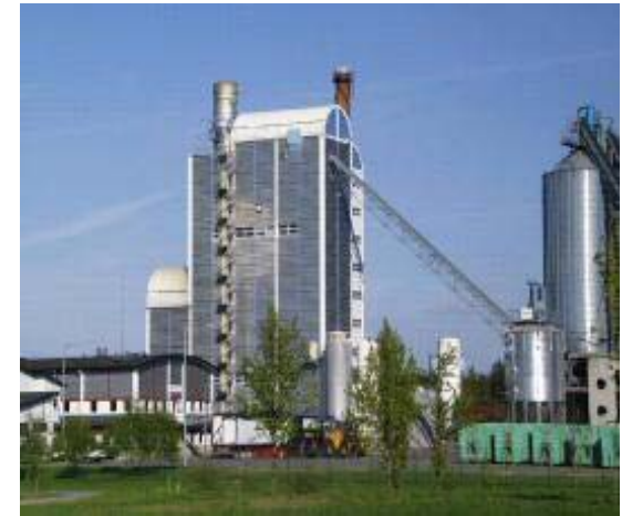
Värnamo, Sweden Integrated Gasification Combined Cycle 6 MWe, 9MWth. CHRISGAS project
