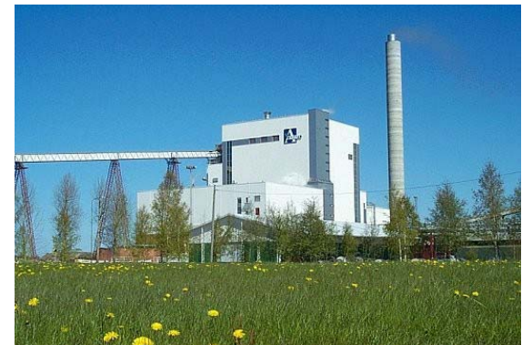
Alholmens Kraft, Finland Combustion power plant, 240 MWe
